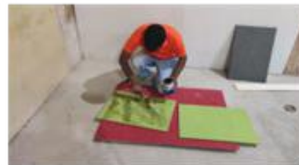
C. Applying adhesive on PET panels
