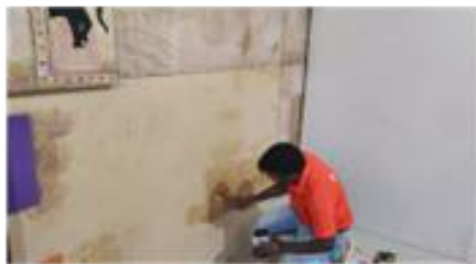
D. Applying adhesive on ply surface
