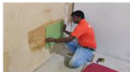
E. Fixing of PET panels on ply surface
