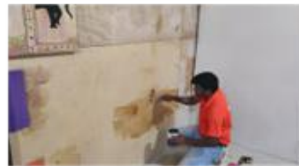
D. Applying adhesive on ply surface
