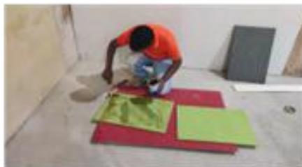
C. Applying adhesive on PET panels
